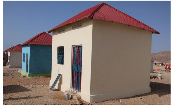
Completed permanent shelters and in Grible-2 Durable Solutions Site in Bossaso. © NRC
