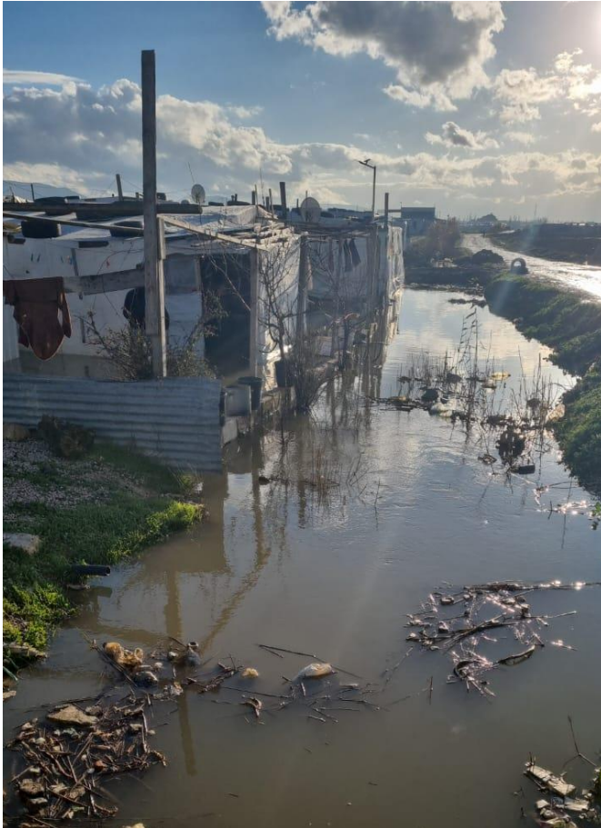
Figure 4. Photo Credit: HAND | Location: Maalaqa, Zahle, Bekaa, January 2024. Flooded Site identified in need of dewatering and floor raising kits.
