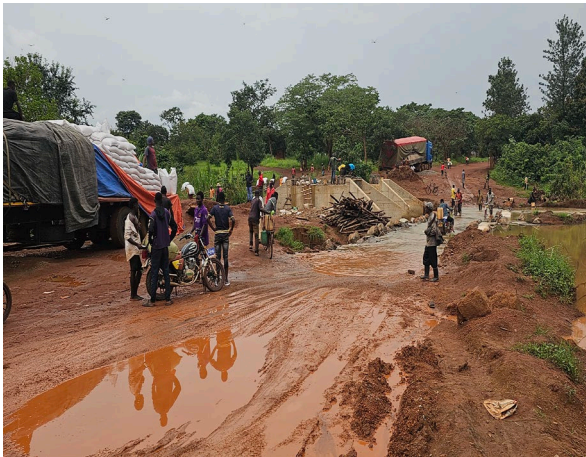
Heavy rains damaged the bridge at the entrance of Nyarugusu Refugee Camp, disrupting services to over 136,000 refugees. © UNHCR/Maimuna Mtengela
