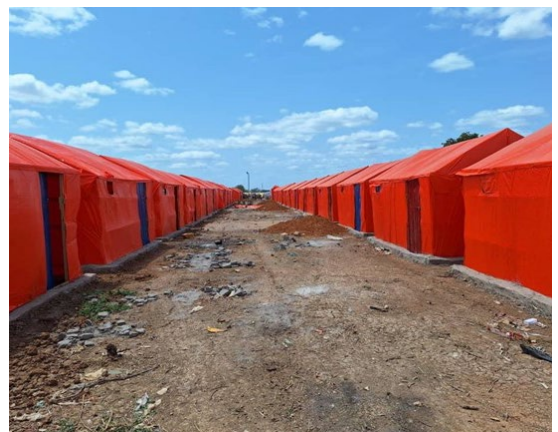
Completed emergency shelters in Bardheere. © AVORD
