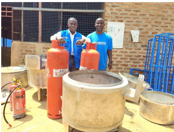
UNHCR installed three clean cooking gas systems at the camps' departure centers and Nyarugusu camp main hospital. © UNHCR/Maimuna Mtengela
