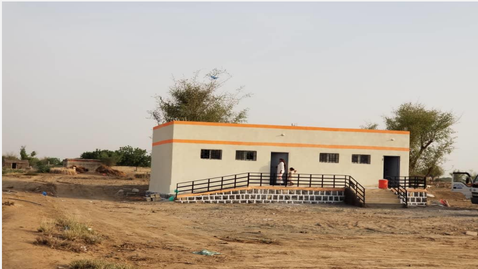
JAAHD The construction of two classrooms in Mehsam Mubara, Al Hodeidah
