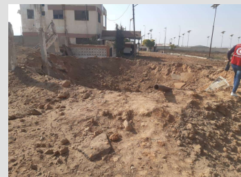
Damage at Joussieh crossing from the recent airstrike | © UNHCR Syria
