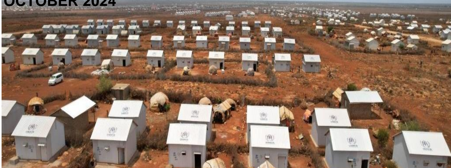
UNHCR Completed the Construction of 194 Transitional Shelters in Baidoa © AVORD
