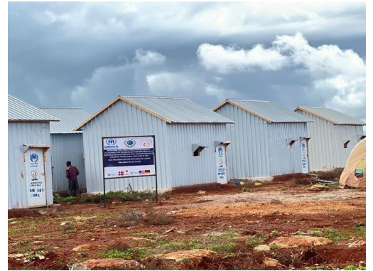
Newly constructed semi-permanent shelters at the Barwaqo-2 Site in Baidoa. © AVORD
