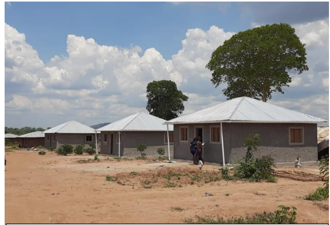
Resilient shelters in the Corrane IDP settlement and in surrounding host communities ©UNHCR Mozambique
