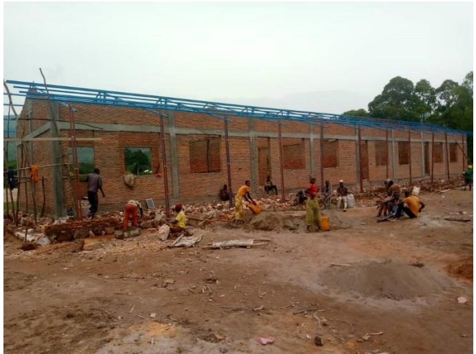
Ongoing construction work at the Butegeri school in Giharo, Rutana Province
