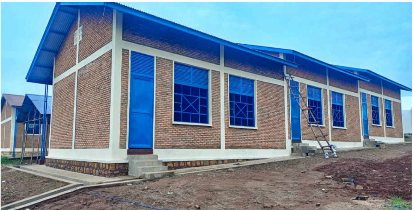
Three newly constructed blocks at the Gitara transit Center in Makamba province. The transit center receives Burundian returnees who chose voluntary repatriation to their home country.
