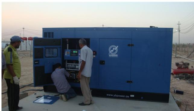
*A 250 KVA capacity generator has been installed in Al-Qaim*
