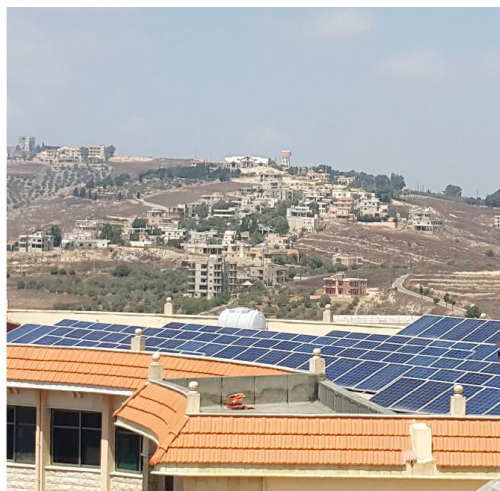
Figure 3 - Installation of a 116 KWp Hybrid - PV Diesel system in South Lebanon Amal Education Institute- Tahrir Square- Sultaniyeh. Photo credits: UNDP
