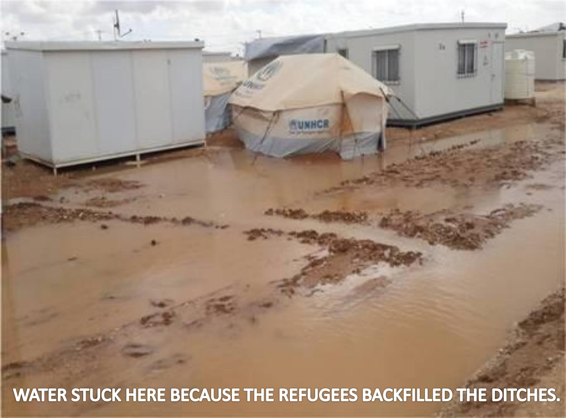
**WATER STUCK HERE BECAUSE THE REFUGEES BACKFILLED THE DITCHES.**
