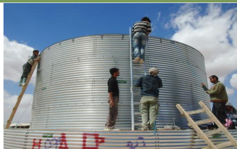
Installing a water tank in Zataari camp, Jordan. Oxfam/Caroline Gluck
