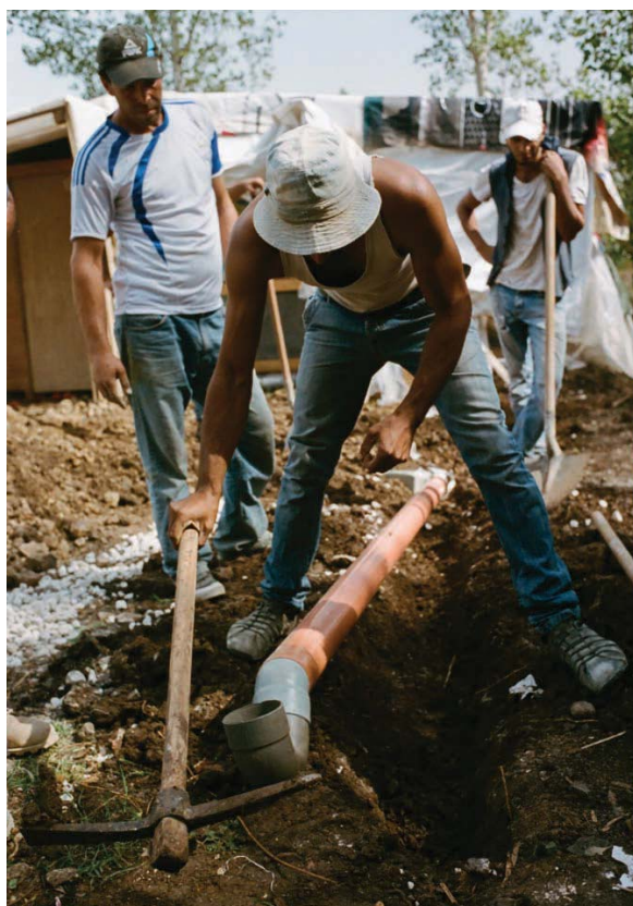
Construction of latrines. Photo credits: James Giles
