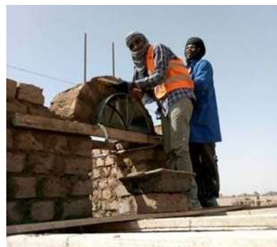
Training in brick construction in Nouakchott. © UNHCR / Mauritania.
