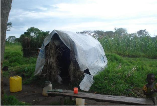
Fig 5.13a: A reed hut covered with a plastic sheet, usually the first housing unit for a refugee. Photo taken by S A K Magezi Nov 2012
