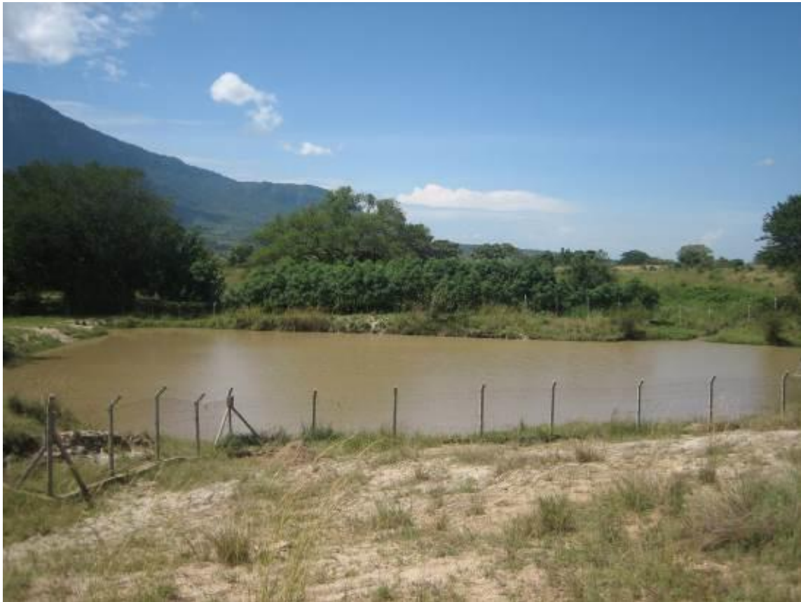
Figure 16: Water dam fenced with barbed wire to keep off livestock and children (Source: FAO/MAAIF, 2013 10 )
