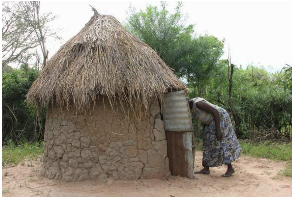
Figure 15: : Mud and wattle pit latrine in rural areas in Palabek areas
