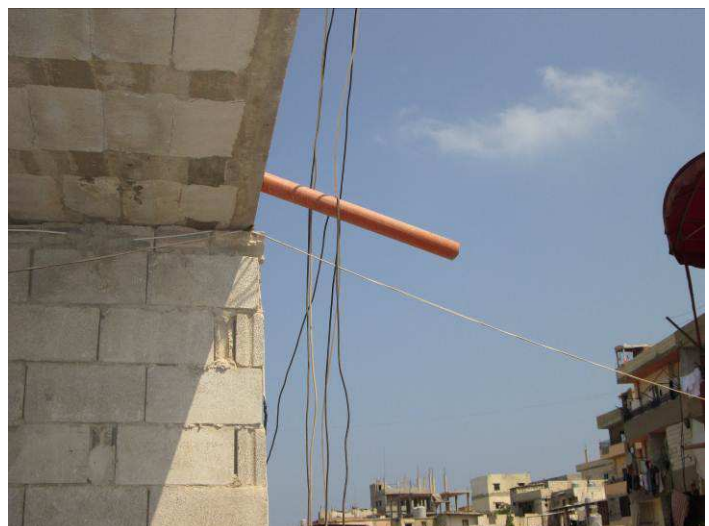
Picture 5: Grey water is discharged directly into the streets
