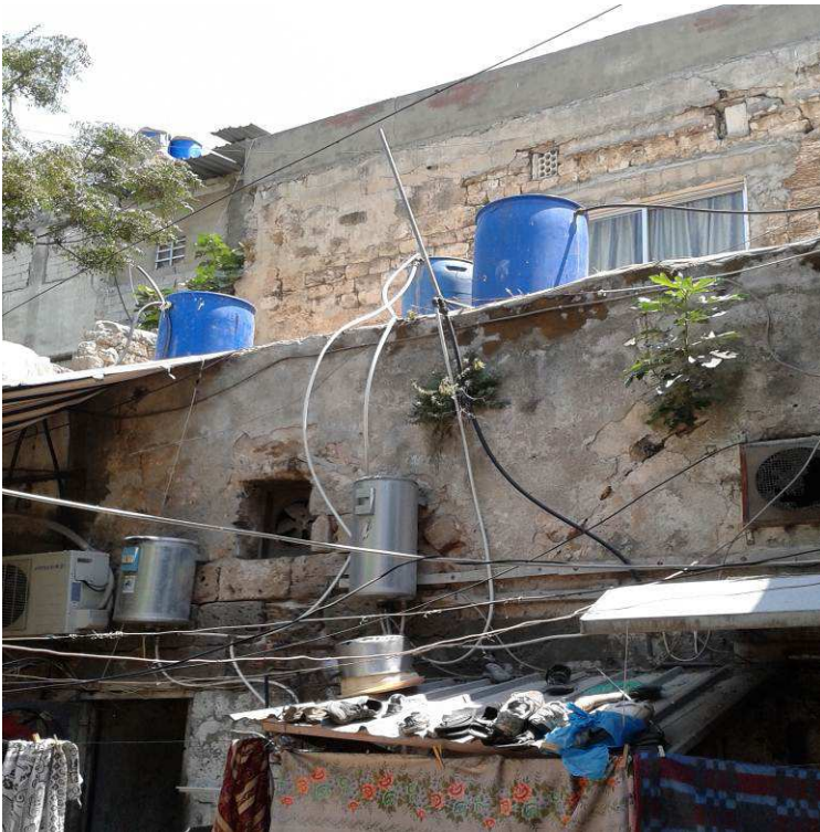
Picture 1: Uncovered water tanks
