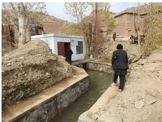
The project involves the construction of a Micro Hydro Power (MHP) plant with an intake, 300 metre feeding canal, forebay, penstock, power house with turbines and gridlines to individual households.
