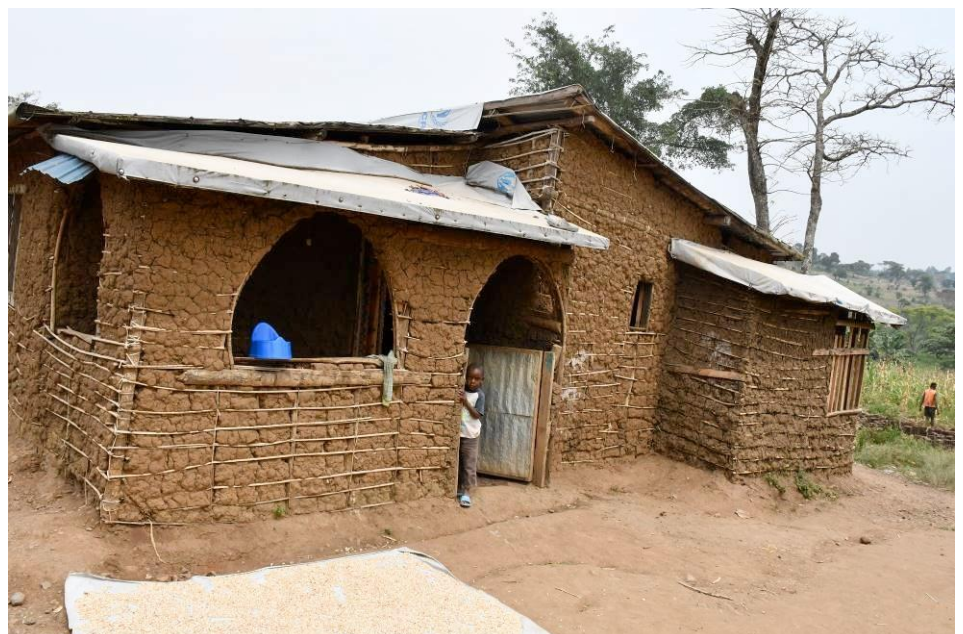
A creatively constructed house by a refugee in Rwamwanja refugee settlement, Kamwenge district. Photo ©UNHCR/Duniya Aslam Khan
