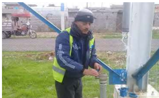
Maintenance of water network in Qushtapa camp, Duhok/UNICEF
