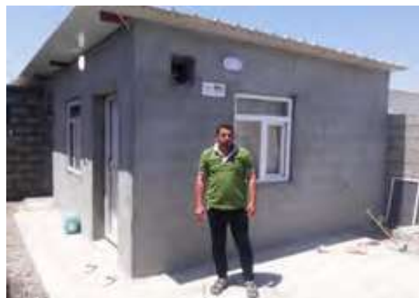
Upgraded shelter in Qushtapa Refugee Camp. Luay Al-Alousi/UNHCR
