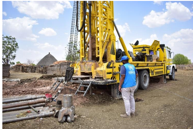
The drilling of a bore hole in Babikri © UNHCR
