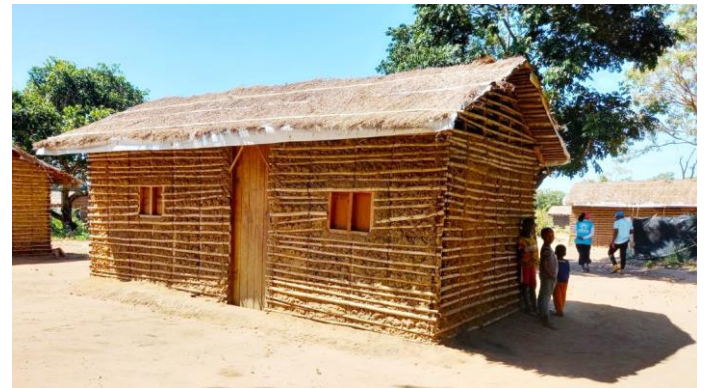
Shelters built by UNHCR and SI in Mueda. ©UNHCR/Irene Matevu
