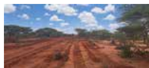
Mirqaan site Clearance (20m width access) ©UNHCR/Silas Omondi
