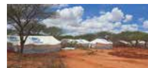
Installation of Family Emergency Tents ©UNHCR/Silas Omondi
