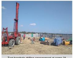
Test borehole drilling arrangement at camp-21 under Teknaf Ground Water Project
