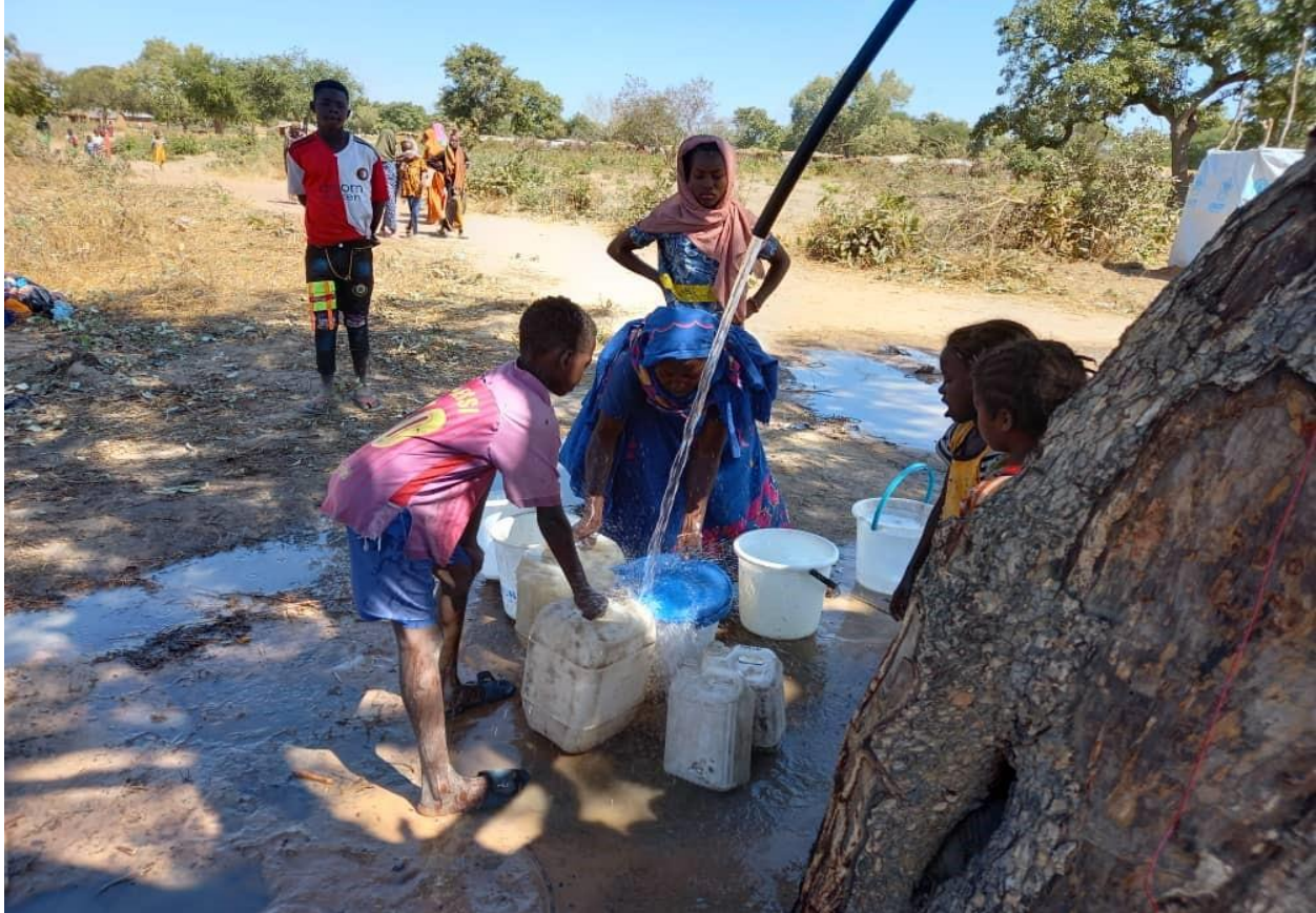
A new water point has been built in Korsi, increasing the supply of water to families. © UNHCR/ Bobo Kitoko
