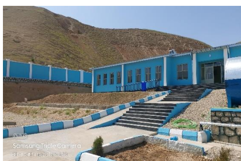
Construction of 8-classroom school building in Sar-Pul City in 2023@UNHCR
