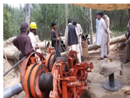
Water supply project in Turkchin village of Sar-Pul City @UNHCR
