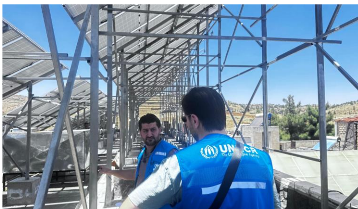
The installation of solar kits at Jdaidet Yabous, ©UNHCR Damascus
