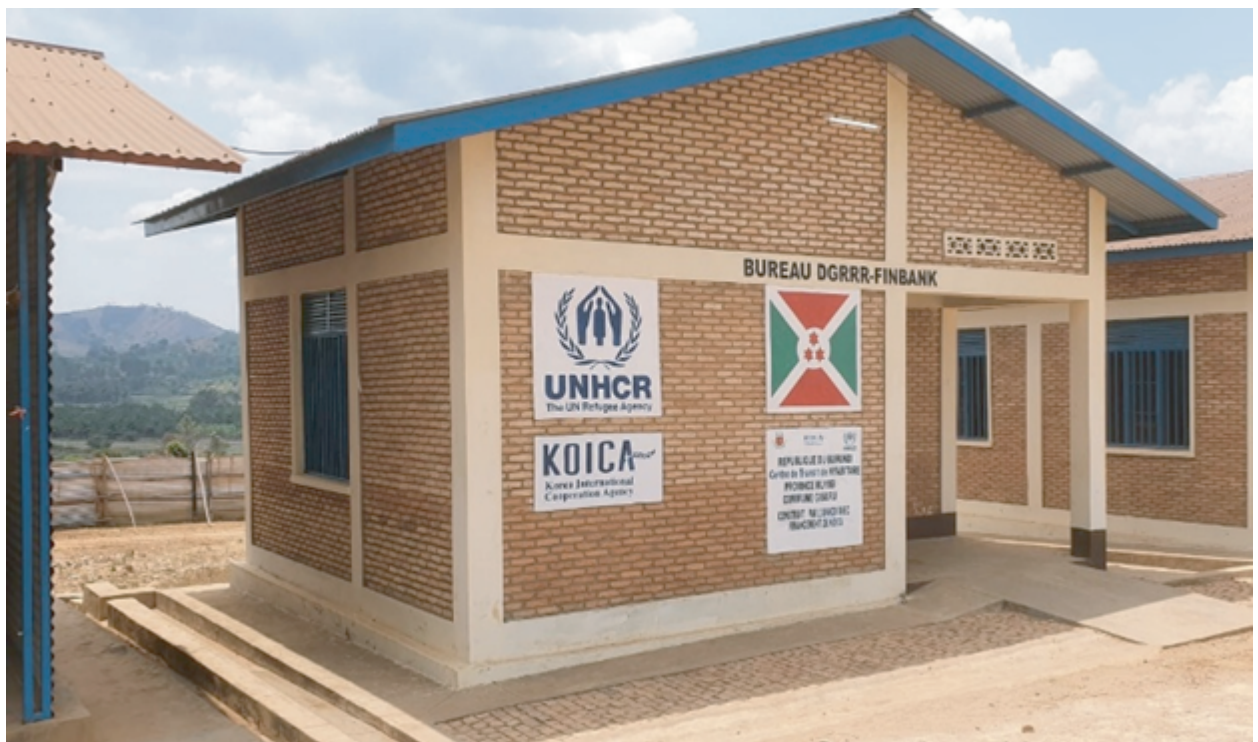
Newly constructed infrastructures at the Nyabitare transit Center funded by KOICA. The transit center receives Burundian returnees who chose voluntary repatriation to their home country. @UNHCR/Burundi
