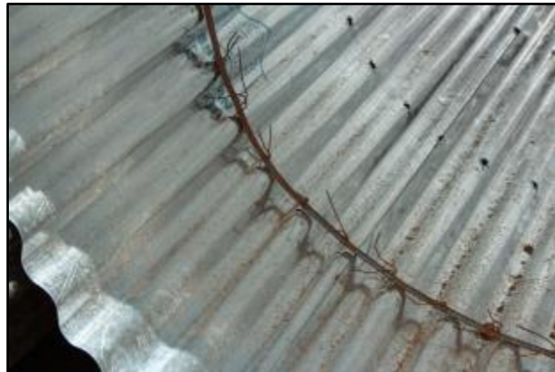
Attachment of the iron bar to the GI sheets
