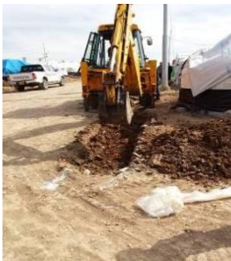
Construction of open channels in Domiz 2@ UNHCR/F.Yousuf
