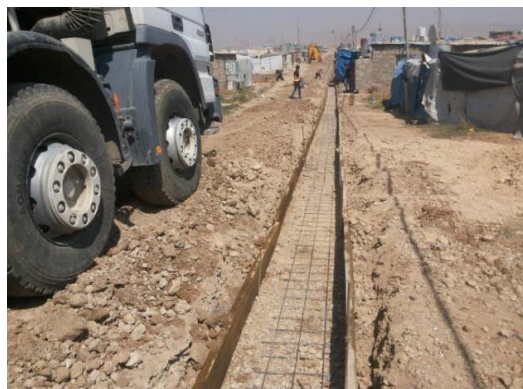
Domiz 1 camp, Construction of open channels. Duhok, August 2015. UNICEF/Abdijabar Khalid
