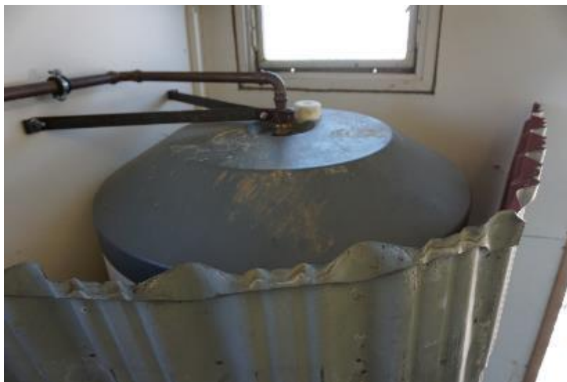
The water heater in the men's shower container – limited volume
