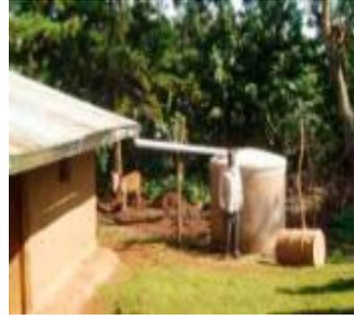
**Picture 6. 12: Ferrocement Tank (4m<sup>3</sup>) in Kapchorwa**
