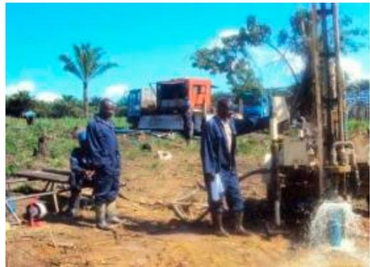
*Picture 6. 9: Borehole drilling and development with a PAT 301 rig and an ELG 15 bar compressor*
