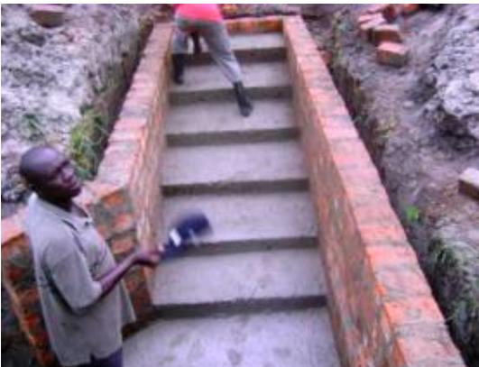
Picture 6. 3:Spring construction in Oyam
