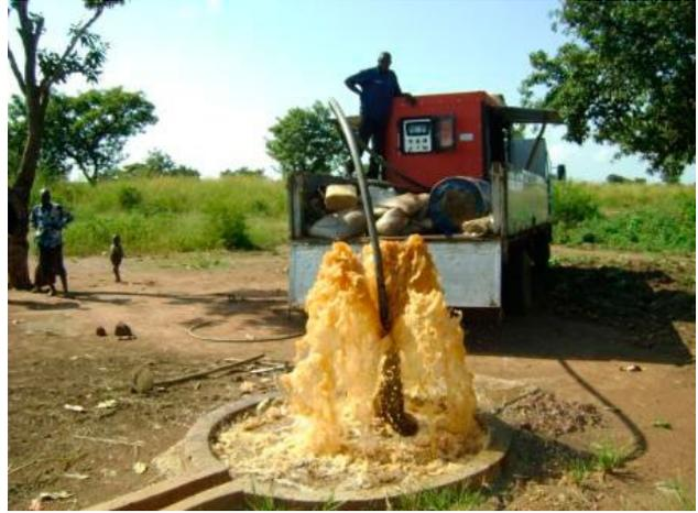
Picture 5. 6: Borehole blowing/cleaning in Pader
