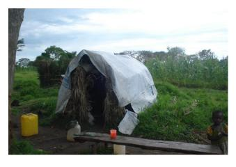
Fig 5.13a: A reed hut covered with a plastic sheet, usually the first housing unit for a refugee. Photo taken by S A K Magezi Nov 2012
