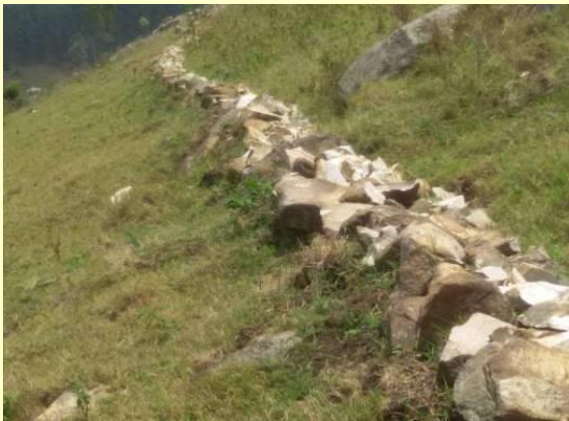
Stone and Soil bunds on steep hill slopes in Rubara Micro Catchment in Rwizi catchment
