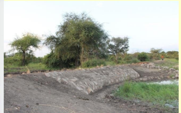
Embankment construction in Aketa dam, Lokok and Lokere catchment
