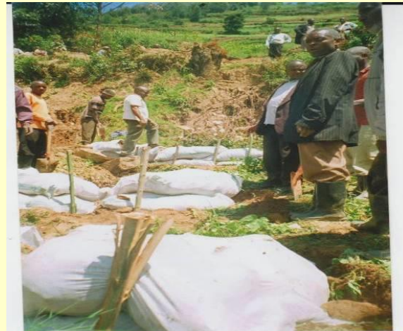
Terracing of steep slopes and gully rehabilitation using sand bags in Rubaya Sub-Catchment
