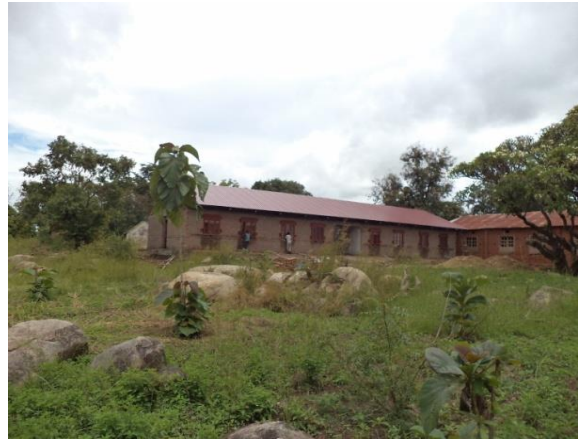
A Dormitory Block being Constructed by LWF PakeleP .S
