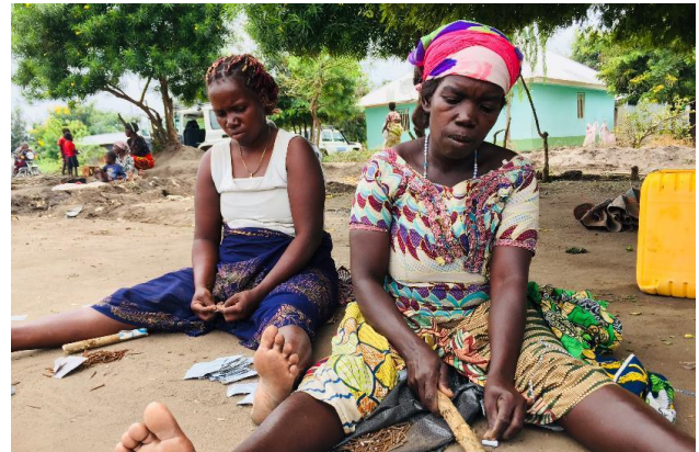
Displaced women preparing materials for the construction of community hangars in a displacement site in Kasenyi, Ituri Province. © UNHCR/Gloria Ramazani
