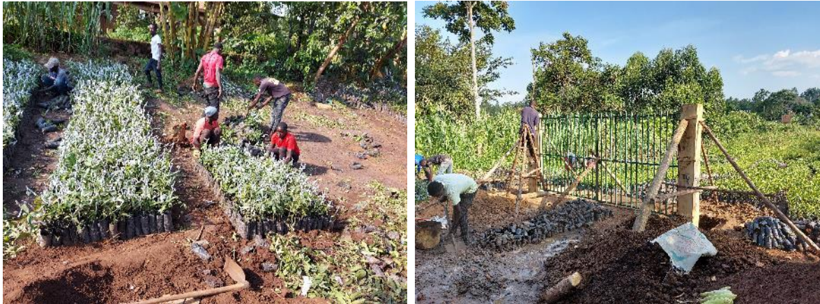
Photo 9: Grafting of mango (left) and installation of gate and fence (right) ongoing at Masindi Nursery
