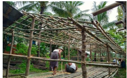
Shelter construction in Central Rakhine. Photo:
