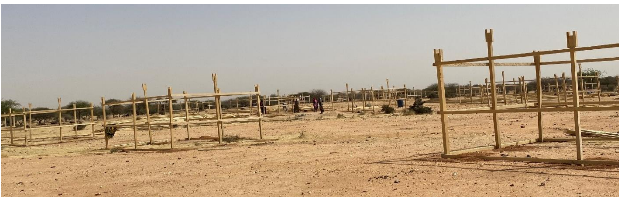
Construction of emergency family shelters in Kouchaguine-Moura camp©UNHCR/E. Umutesi
