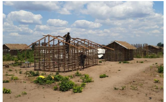
Shelters under construction in Mueda District, Cabo Delgado ©SI
