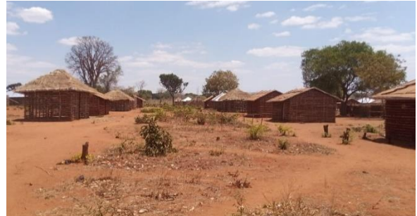
Shelters under construction in Chimoio IDP site, Montepuez. ©AVSI
