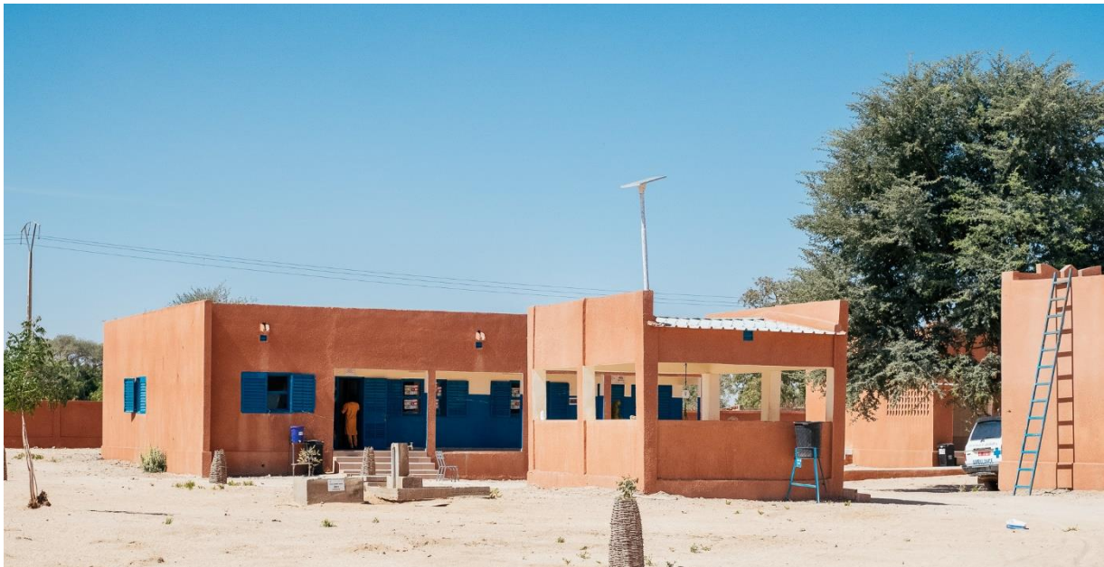
Integrated health centre built in the village of Dan Dadjji Makaou. UNHCR /Romain_Pichon-Sintes
