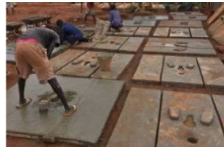
Photo by JAM team; slab production for latrine
