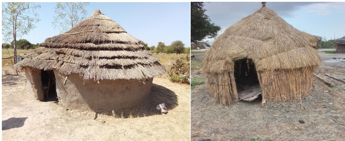
Figure 6: Houses in Aweil 1
