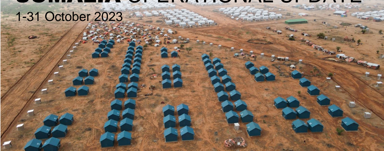
UNHCR, through its partner, completed the construction of 192 transitional shelters (the dark blue houses in the foreground) and 18 latrines at the Ladan IDP Site in Dollow. © AVORD
