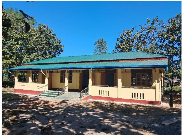
Construction of a community hall as part of a community-based project in Hlaingbwe Township, Kayin State. © UNHCR/Nan Khin
