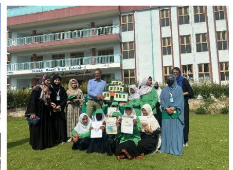
Three Story school building constructed benefiting mainly girls @UNHCR
