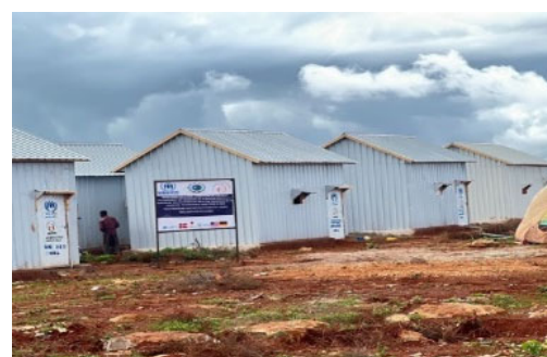
Newly constructed semi-permanent shelters at the Barwaqo-2 Site in Baidoa. © AVORD
